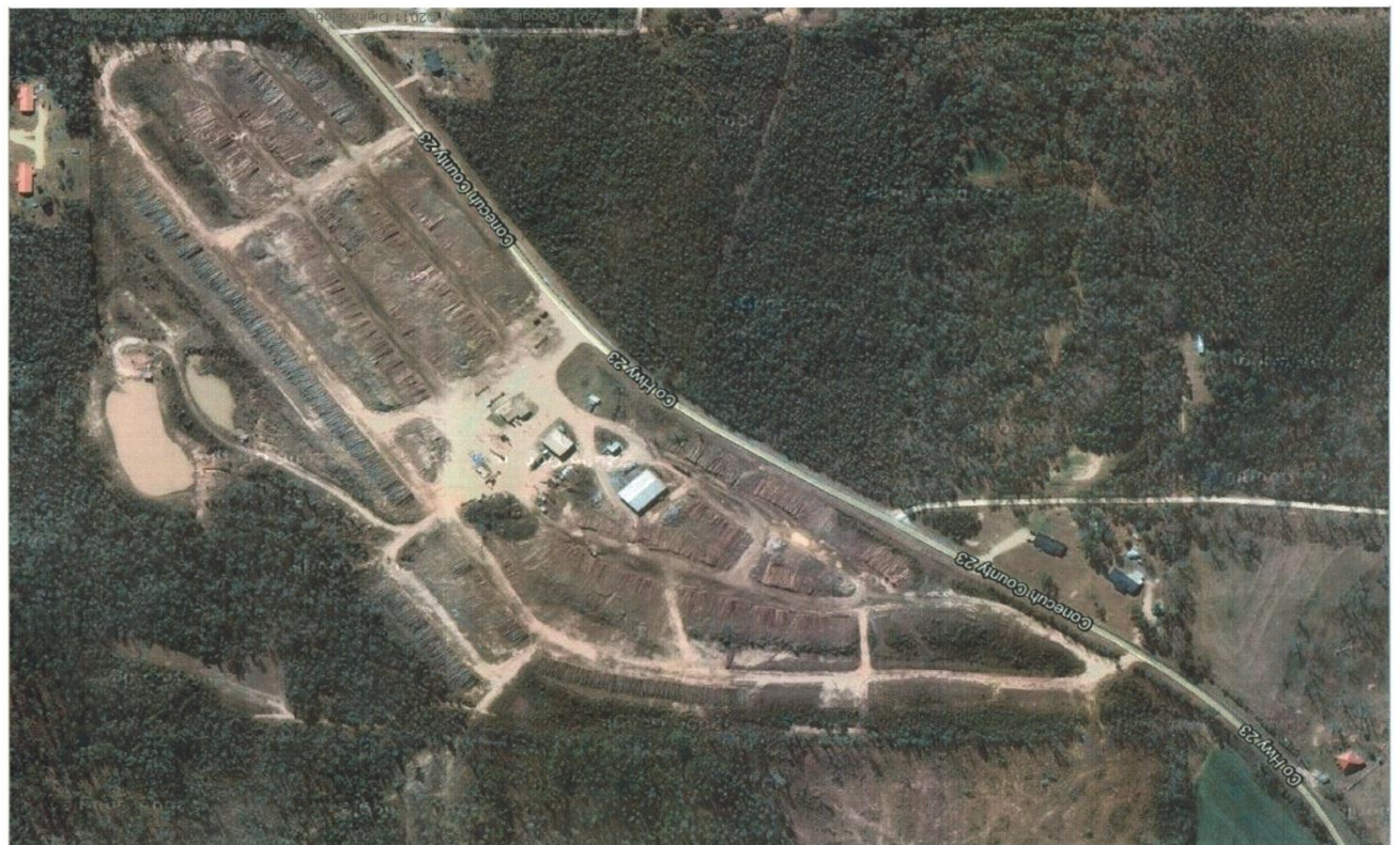
GEC Planta de compostaje Castleberry, Alabama
